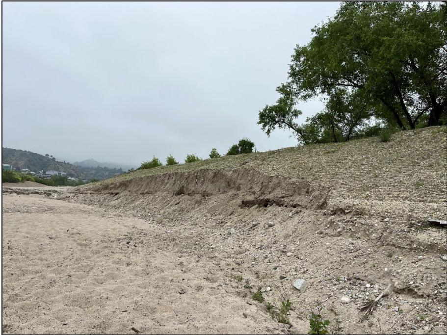
Photo 12: Overview Side Slopes
