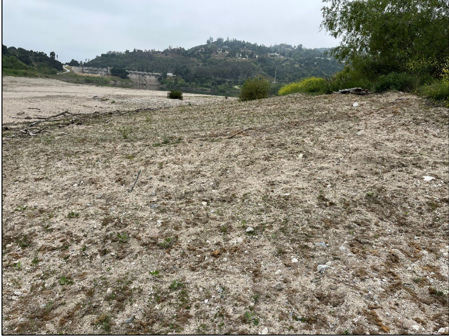
Photo 11: Overview Side Slopes
